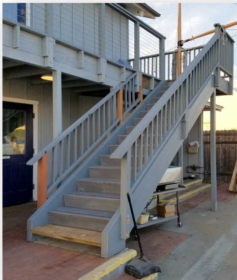
Stair nearly complete and prior to the ministrations of Joe Huntsinger
